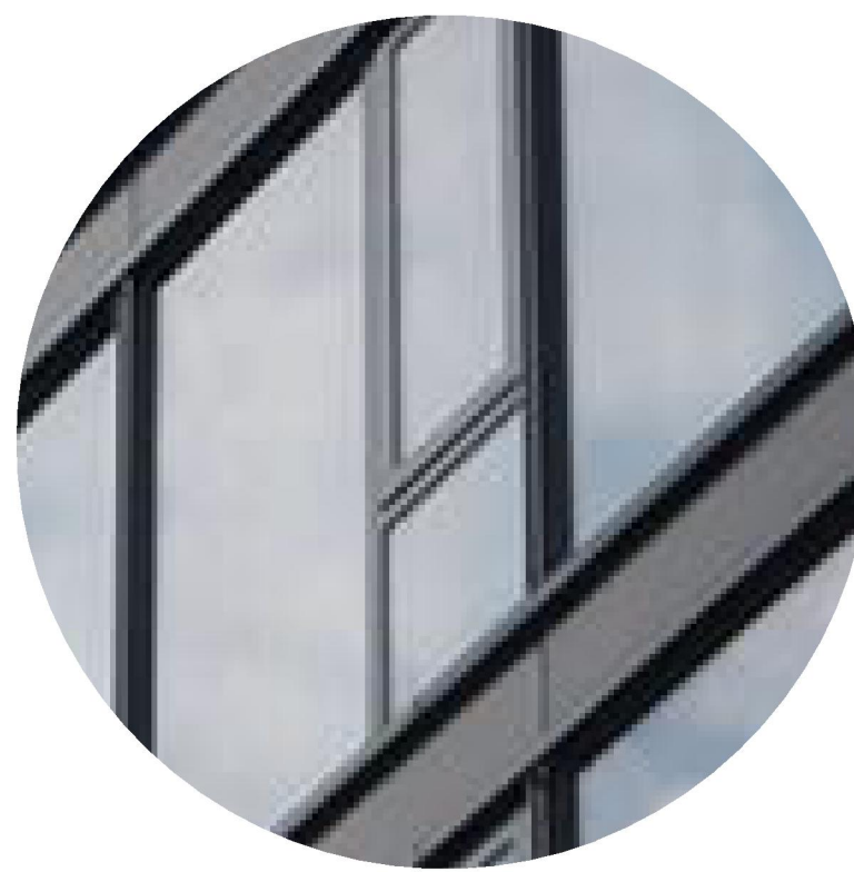
4 TINTED GLASS FOR STOREFRONT / WINDOWS / BALCONY DOORS VIRACON OPTIGRAY
